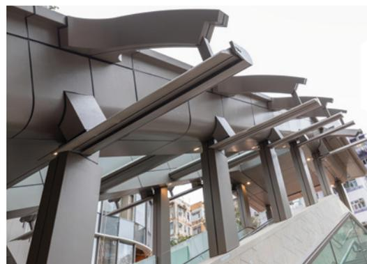
The Air Induction Units installed at Yue Man Square Public Transport Interchange help improve airflow while consuming less energy.
