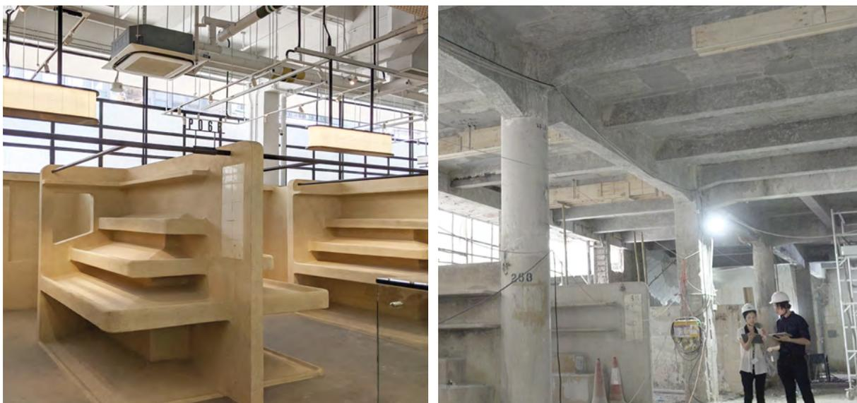
A clear height of over 2.9m was achieved for most areas within Central Market through intensive design and construction coordinations made possible with the BIM tool.
